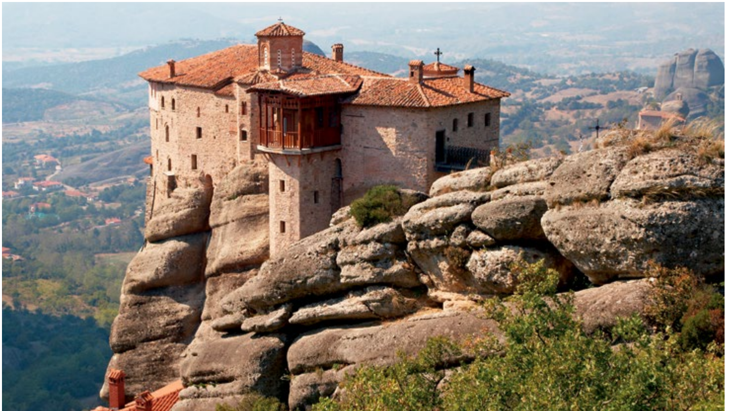
Monasteries at Meteora, Greece
